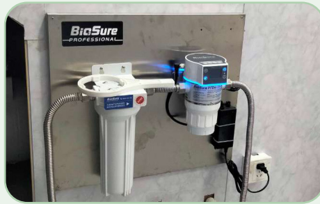
Preventive Maintenance of Water Lines
